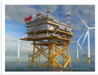
Offshore substation (OSS)
